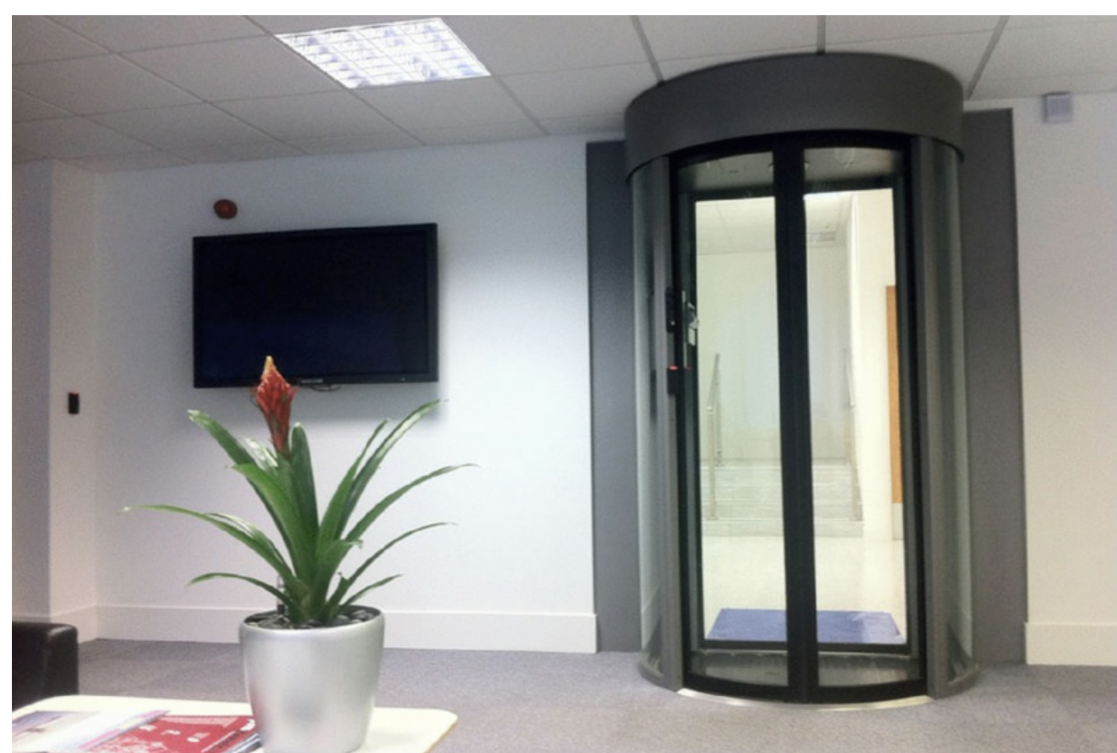
Figure 19.2 A mantrap installed in a lobby
